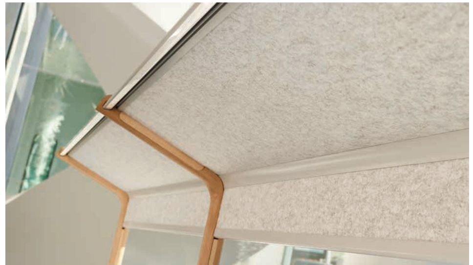
A solid wood Y-frame with LED lights creates an overhead umbrella, trapping sound as it naturally travels upward
